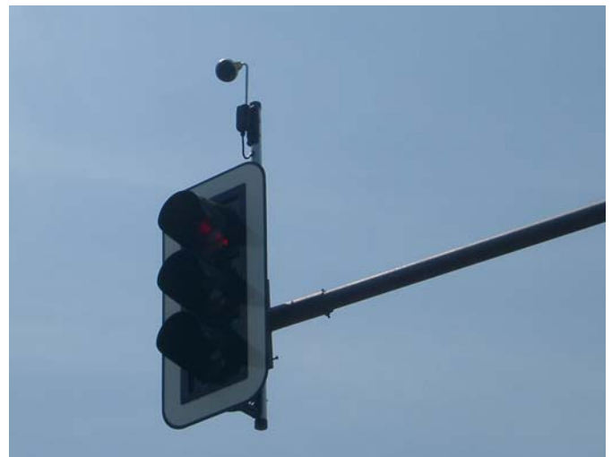
This above-ground sensor allows quick and flexible installation.
